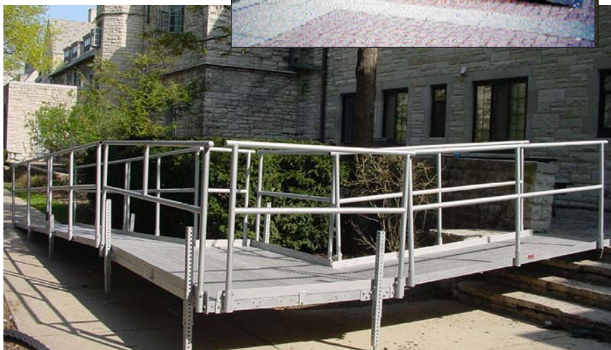
Above: The 'L' shape configuration includes a turning platform and double bar handrails.
