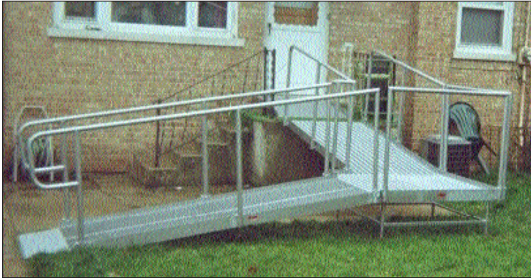
Above: Galvanized Steel Ramp System with plat- forms for home access
