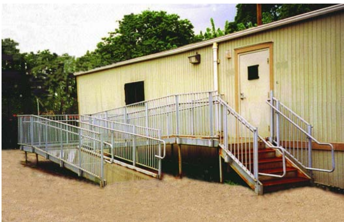
Concrete Ramp System: A modular class room using a 30-foot ramp system with a 180° turning platform and a resting platform and stairs at the entryway door. Handrails are fitted with vertical pickets.
